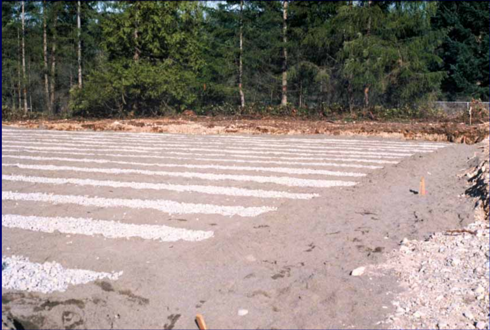
Large gravel bed converted to trenches to provide side walls
